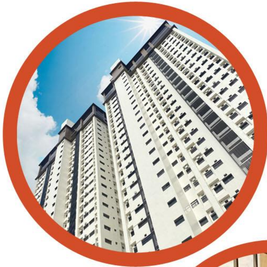
Exterior Photo of Towers 1 & 2
